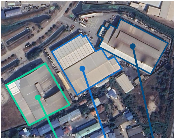
Factory 3 Factory 2 Factory 1
